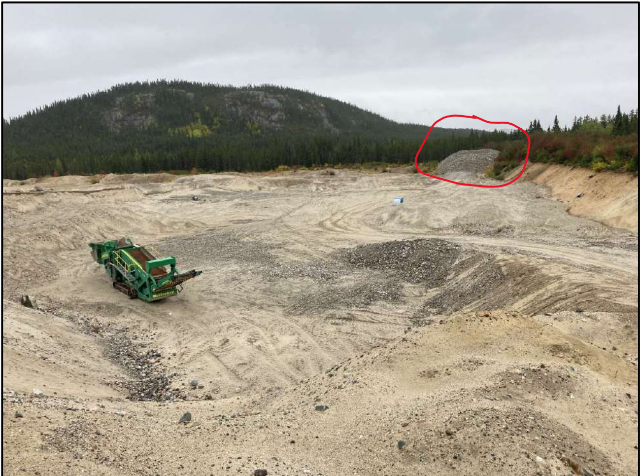
Figure 26: View of the sand pit and pile of pebbles and rocks to be used (2020-08-29)
